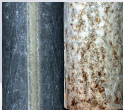
Magnelis® ZM310 welded and re-protected
